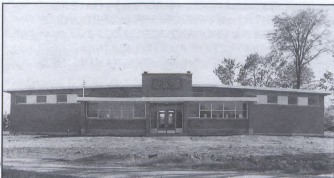
The third Blackburn Public School was built in 1954 and additions added in 1960 and 1963.
