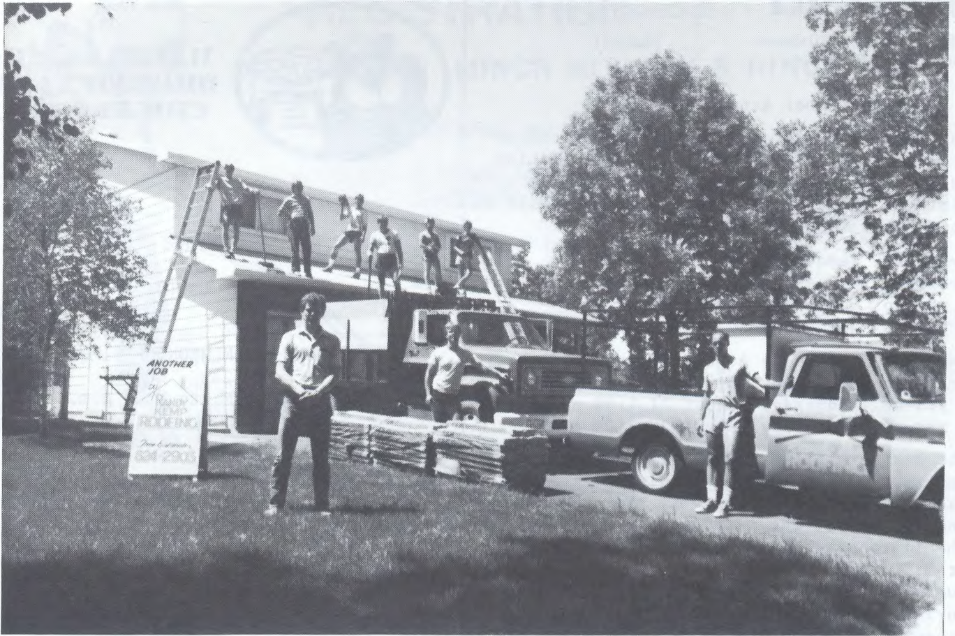
RANDY KEMP AND HIS ROOFING TEAM
